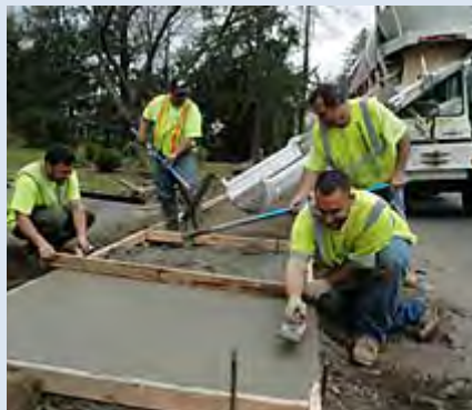
Main Street Sidewalk Construction
