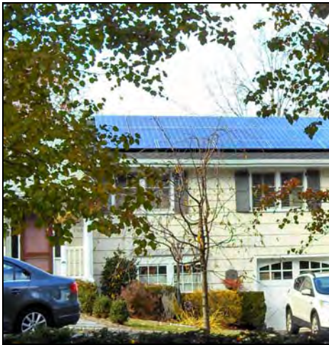
Residential Solar Installation
