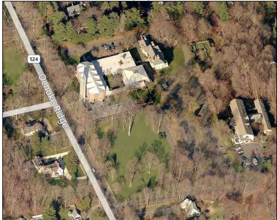
St. Marks Episcopal Church
