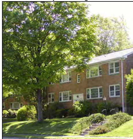
Multi-Family On Heritage Hill Road
